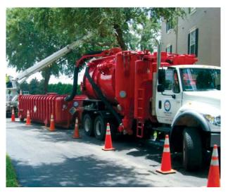
A vacuum truck bypasses its tank and pumps straight into the vacuum container, keeping the vacuum truck at the site working while vacuum containers are filled and hauled away.
